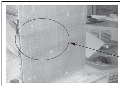
Remove 2 Sheet Metal Screws From Each Side of Coil Assembly
