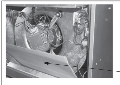
6. Remove the 3 sheet metal screws which attached the blower to the blower shelf located in the air handler control box. (3/8" Socket)
