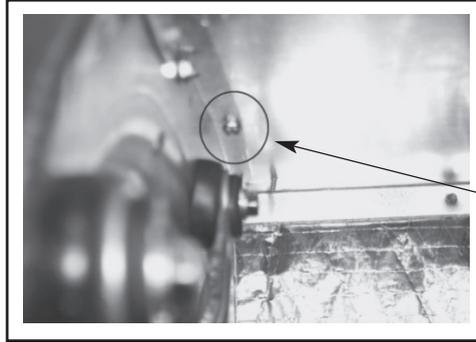
Remove Sheet Metal Screws From Each Side of Blower
