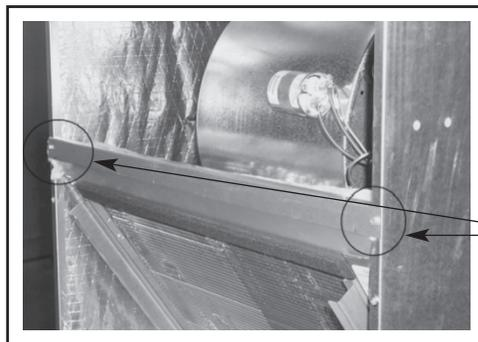
Remove 2 Sheet Metal Screws From Middle Brace
