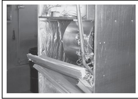
10. Remove the 2 sheet metal screws that attached the blower to the bottom of the blower shelf. (1/4" Socket)
