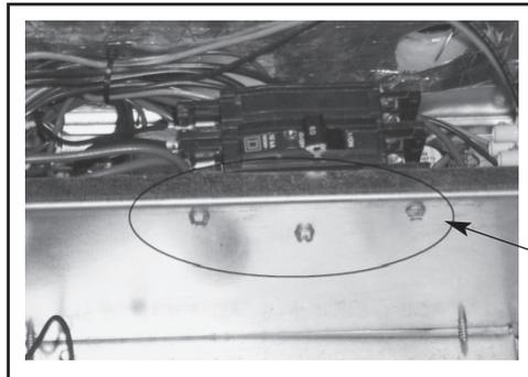
4. Remove capacitor to help prevent damage to the coil. (1/4" Socket)
